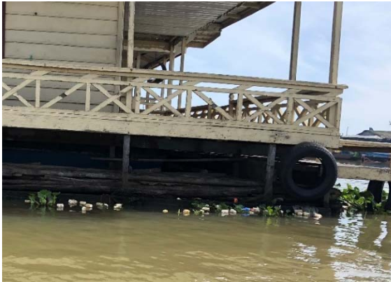
Figure 4 : scuttered plastic waste I
