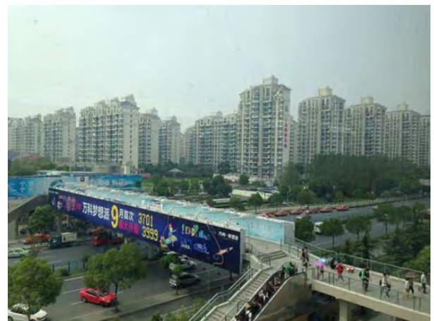
Fig. 12 State of Songjiang College Town Station
