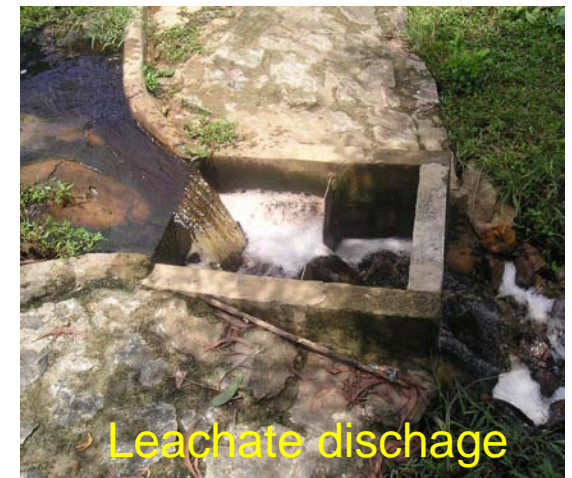
Leachate treatment system
