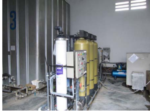
Tap water was treated with ion exchange resins to provide water for cleaning.
